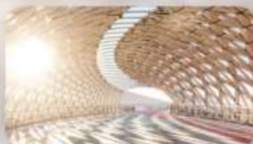
Atyrau Bridge Astana
